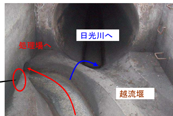
(No.6雨水吐き室内写真)
