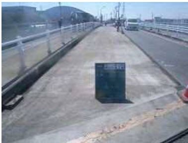
舗装撤去後・防水前
