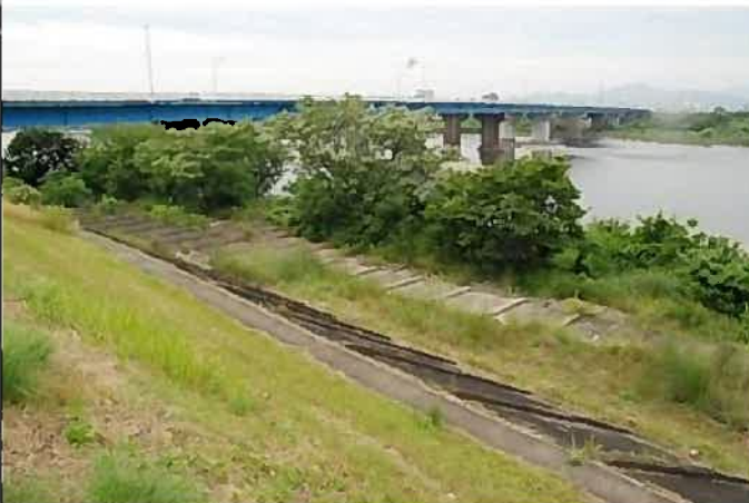
Image 1.3.4: Installed revetment along Kiso River
